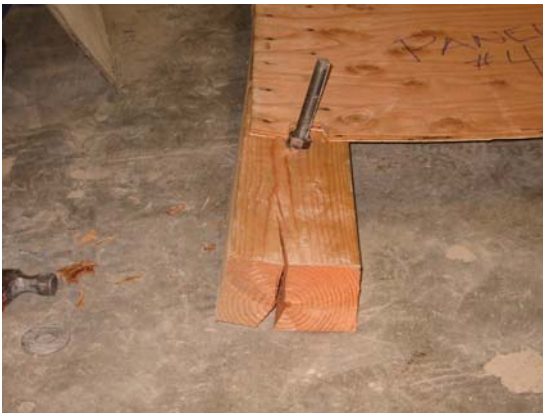
Cross Grain Bending of Top Plate Photograph 6
