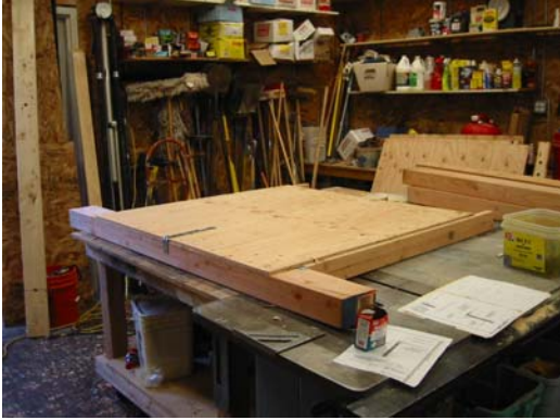
Construction of Test Panel Photograph 1
