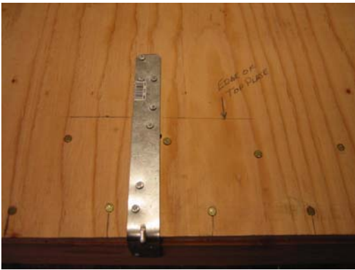
ST12 Strap Installation Photograph 2
